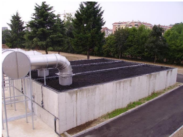
Figure 1 - Mónafil Installation in Milan, Italy
