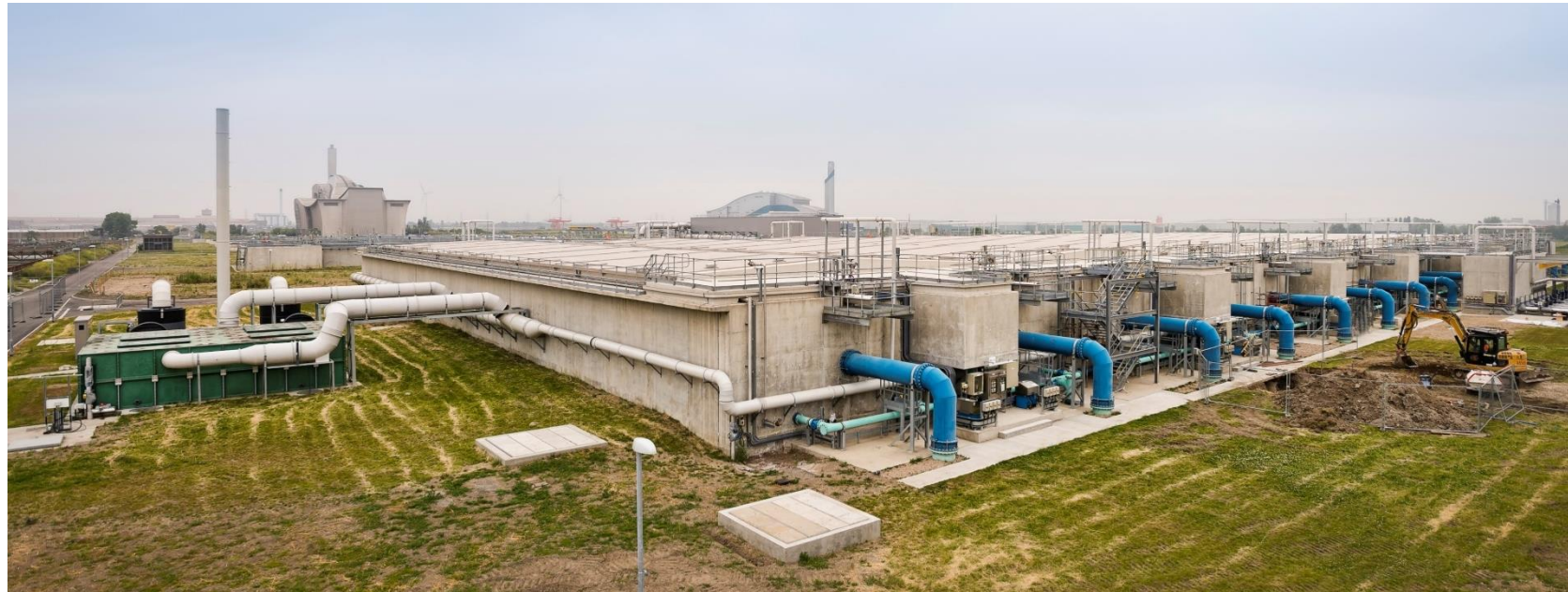
Figure 6 - Mónashell OCU installed in Becton WWTP, London
